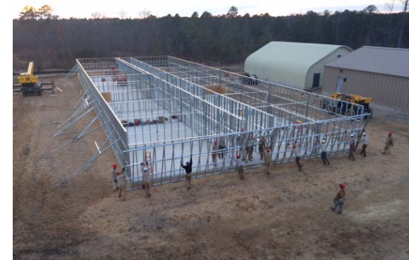
On-site frame and truss manufacture demonstration – Ft. Bragg
