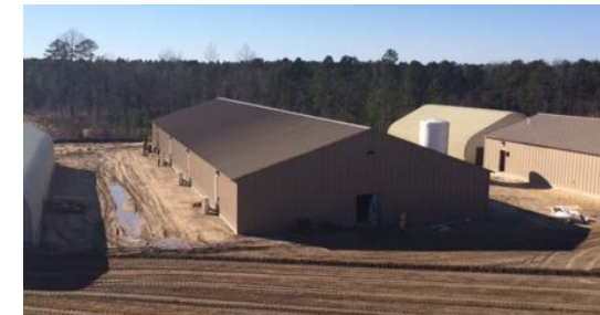
Finished demonstration structure
