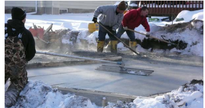
Cold weather concrete
