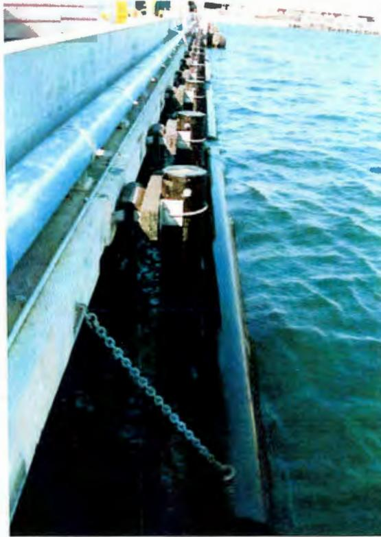
Figure 3: Plastic Fender Pile System
