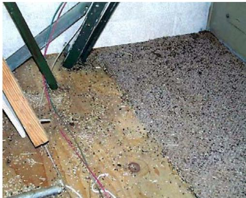
Figure 4. Heavy rodent contamination.
