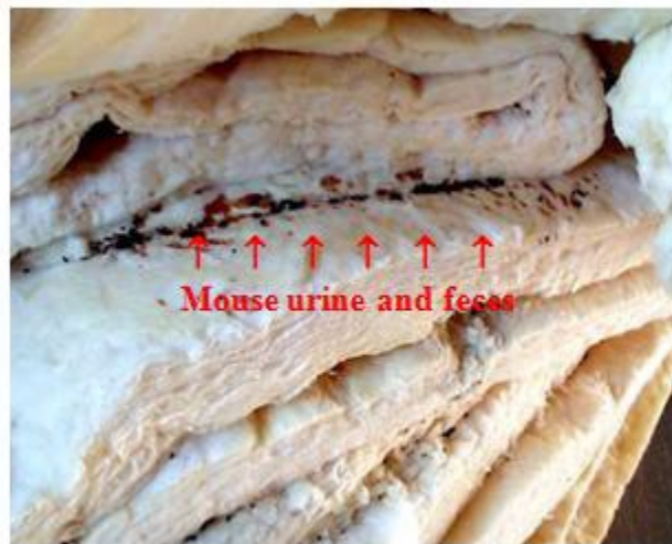
Figure 2. Mouse urine and feces on insulation.
