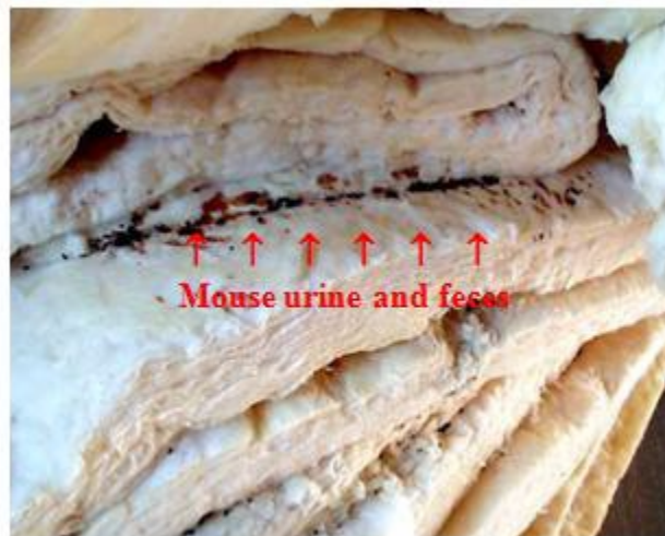
Figure 2. Mouse urine and feces on insulation.
