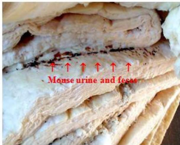
Figure 2. Mouse urine and feces on insulation.
