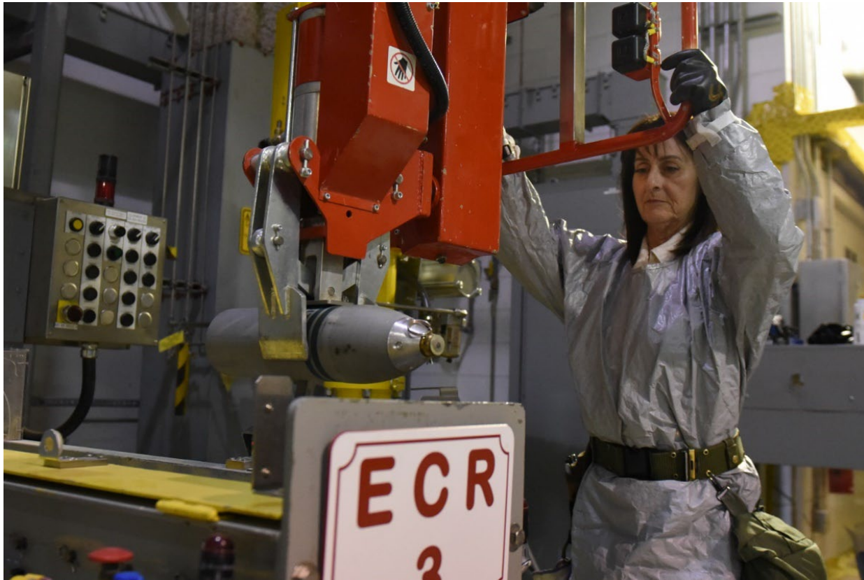
A Pueblo Chemical Agent-Destruction Pilot Plant ordnance technician uses a lift assist to transfer a 4.2-inch mortar round onto a conveyor for its destruction in spring 2023. Conveyors transported munitions into Explosive Containment Rooms, where energetics were removed before chemical agent was drained and neutralized.
